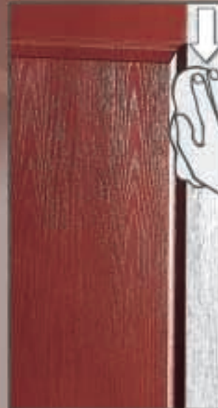
Use a clean rag to remove accidental staining from areas not due for immediate staining.
